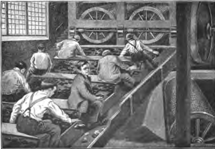
A Coal Breaker.
